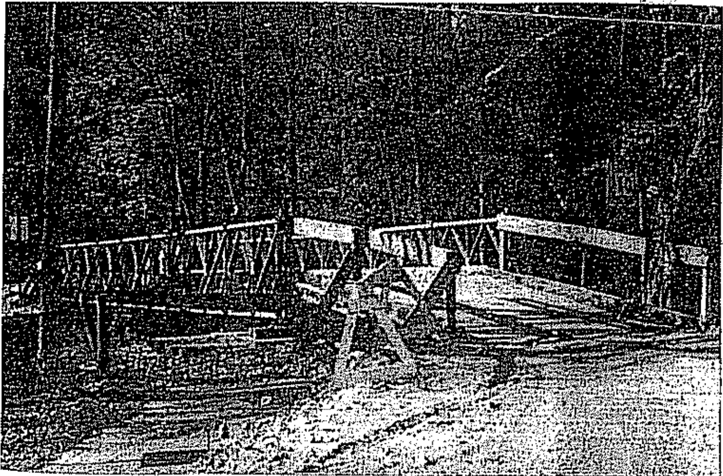
SOUTHAMPTON—A temporary bridge over the west branch of the Manhan River at Russellville has been erected by the state DPW. The Bailey Army surplus bridge is about 50 feet long with ramps on either side to allow passage of one vehicle at a time. Local truck
